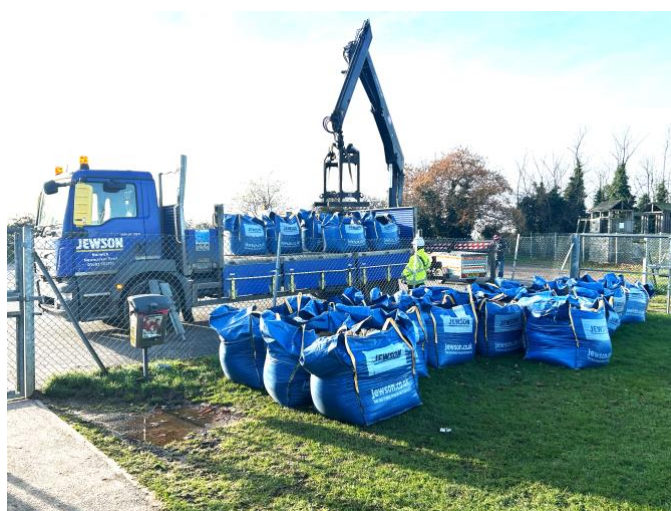
Ballast, sand and pea gravel being delivered
