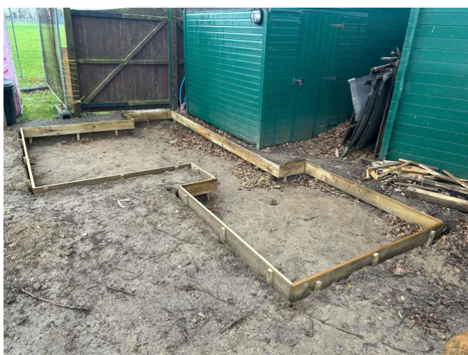
Shuttered foundation for the Toilets
